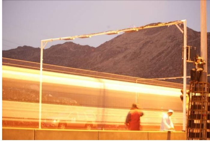
Fig. 6. The RFID readers installed at Arafat entry
